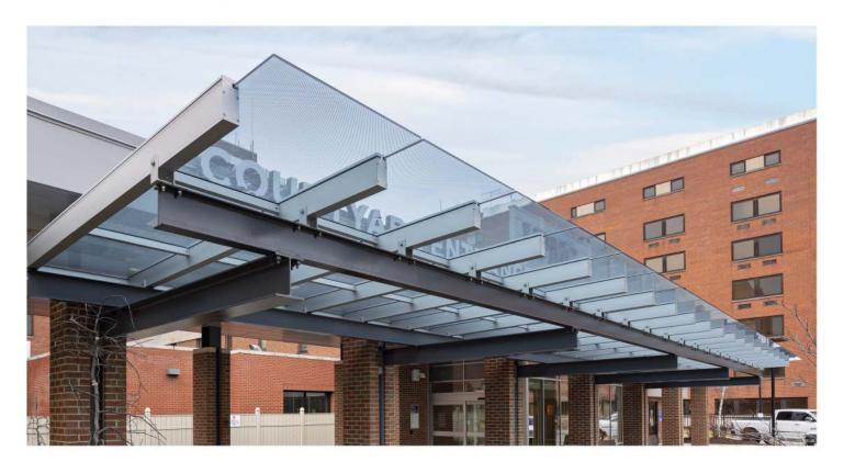
The SKYSHADE 2500 is a sleek, long spanning glass canopy system that incorporates continuous mullions, which secure the glazing. An internal gutter system, sturdy aluminum framing, and full fabrication are just a few benefits that the SKY-SHADE 2500 system has to offer.
