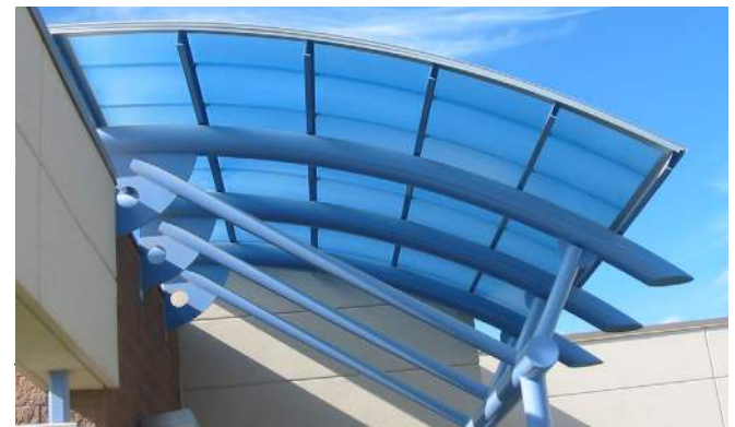
SKYSHADE entrance canopy at a school in AZ
