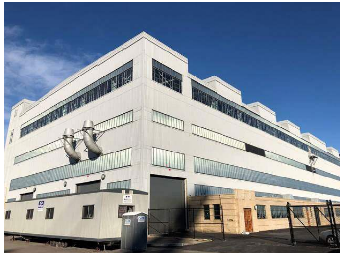
LIGHTWALL system with custom mullions for century old warehouse
