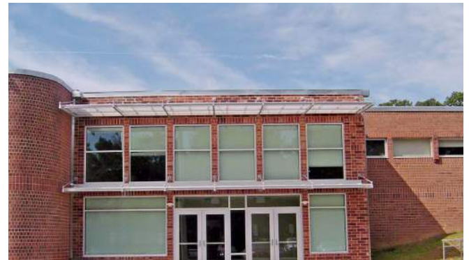
SKYSHADE® Canopies at NC National Guard Readiness Center
