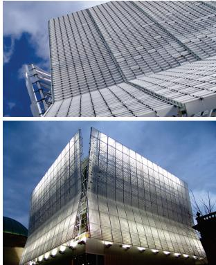
KINETICWALL® is a dynamic façade system comprised of flappers that move with the wind, creating an eye-catching and unforgettable aesthetic.
