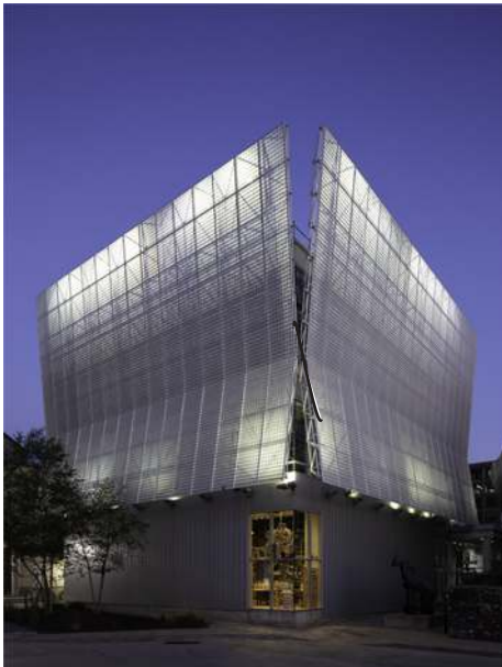
EXTECH's KINETICWALL at the LEED certified building, The Children's Museum of Pittsburgh
