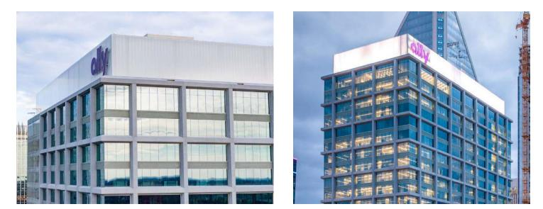
LIGHTWALL 8000 translucent polycarbonate system is ideal for screen applications, capable of long spans with minimal structural support. The system provides a continuous screen, specifically beneficial for backlighting applications where shadows from the supporting structure are a concern.
