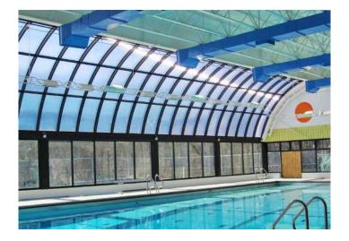
The SKYGARD 3300 is a commercial skylight system with aluminum mullions that can fit a variety of glazing panels and widths. This flexible, non-structural 'skin' system is designed primarily for monolithic or cellular polycarbonate glazing, although glass can be used.
