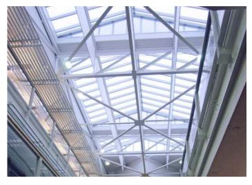
support. It is ideal for over-glazing or retrofit applications where existing structural members will remain in place.
