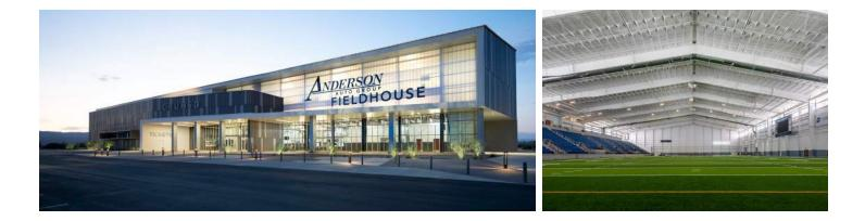
The LIGHTWALL 3440 is our most popular daylighting system. The 3440 system offers beauty, durability, and economy with vertical panels that can extend up to 54 feet long and eliminate leak-prone horizontal joints.
